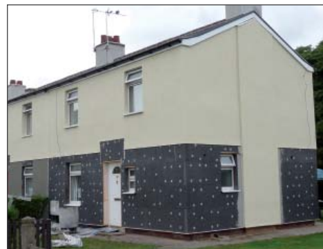
Insulation boards fixed to property, first floor completed with acrylic finish.
