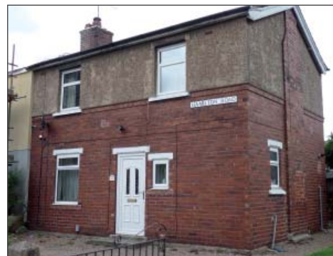
Dorman Long property before the installation of external wall insulation.
