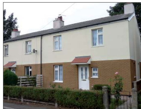
Completed house with light cream acrylic render to the first floor and brick effect render, with golden buff brick face and charcoal mortar layer, to the ground floor.
